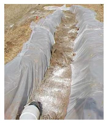
The ditch was made with two rows of straw bales covered with plastic and lined with two layers of an open-weave jute matting sprinkled with the appropriate Silt Stop<sub>®</sub> powder.
